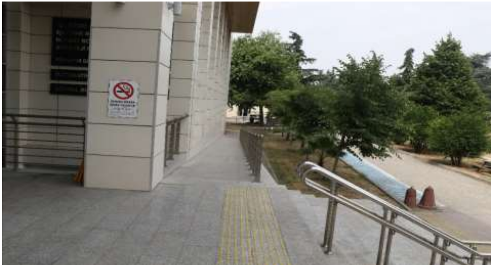
Pedestrian path for disabled pedestrian (faculty buildings entrance)
