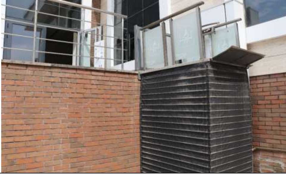
Disabled ramp for disabled pedestrians
